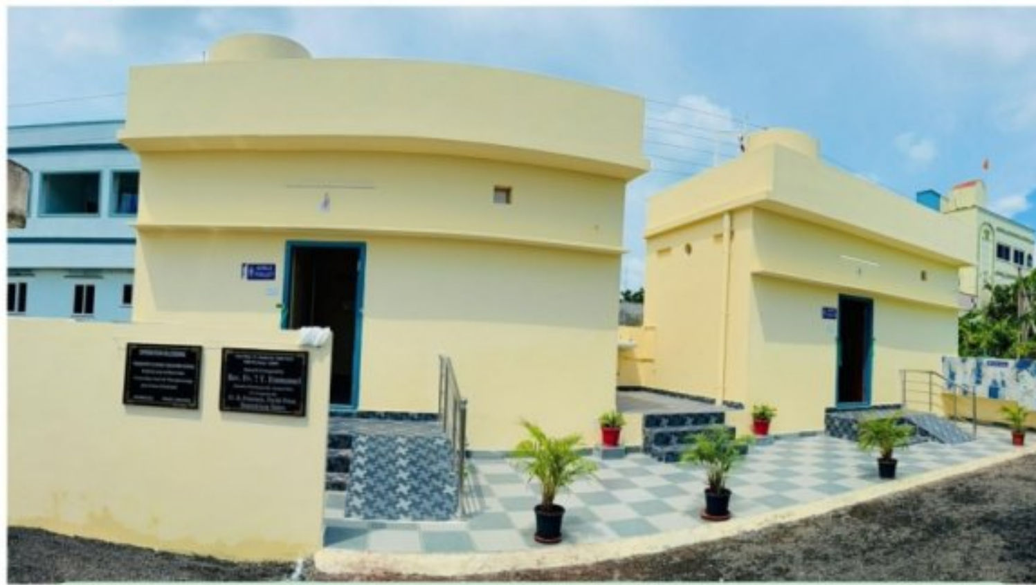
IJEMHS, Bhuvanapalli - Toilets Block
